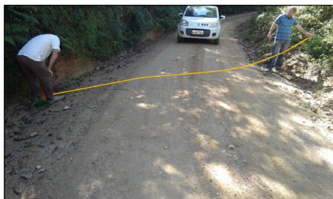
Figure 4. Checking the required length for a culvert.
